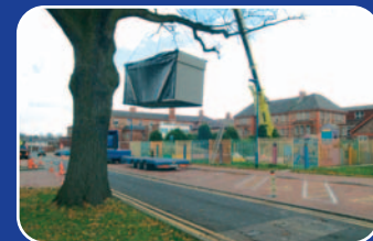
At the end of November the Unit was dropped into place
