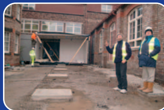
November 2003: The ground was prepared for the installation of the unit
